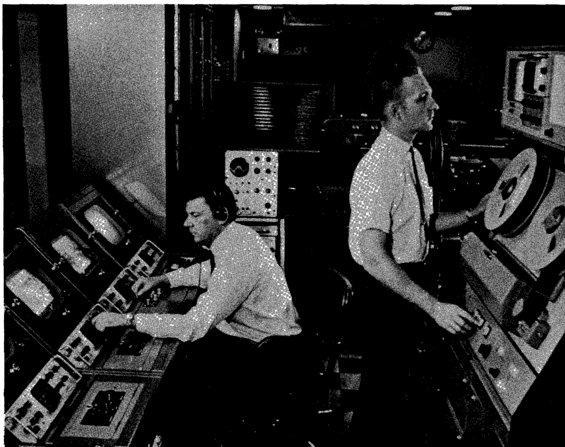
NMAC television control room.
